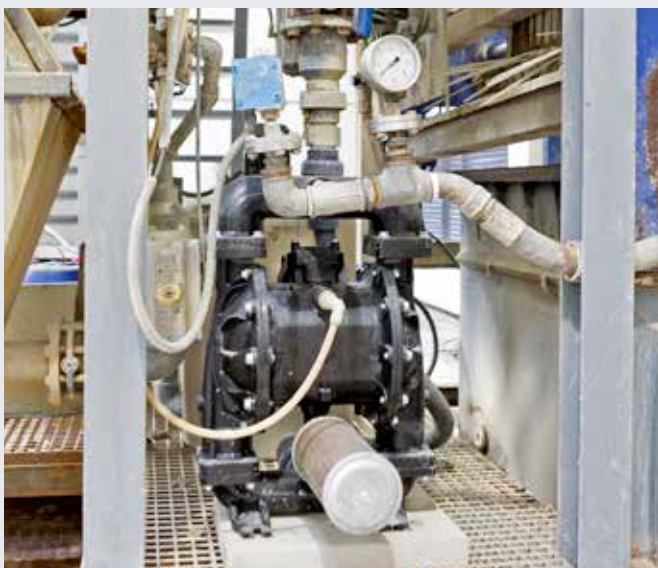
High suction lift reduces pump delivery.
