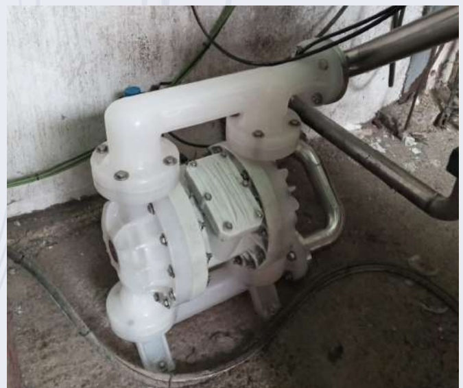
High fluid viscosity reduces pump delivery.
