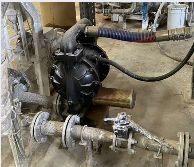
High suction lift reduces pump delivery.
